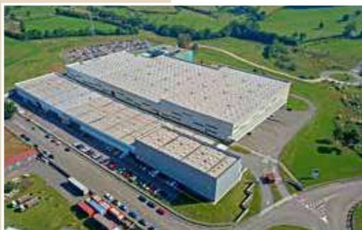
Research & Development and Manufacturing facility in Gijón (Spain)
