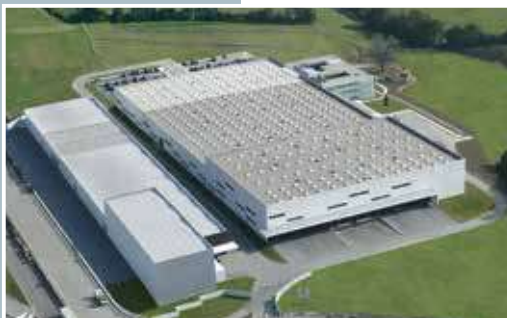
Research & Development and Manufacturing facilities in Gijón (Spain)
